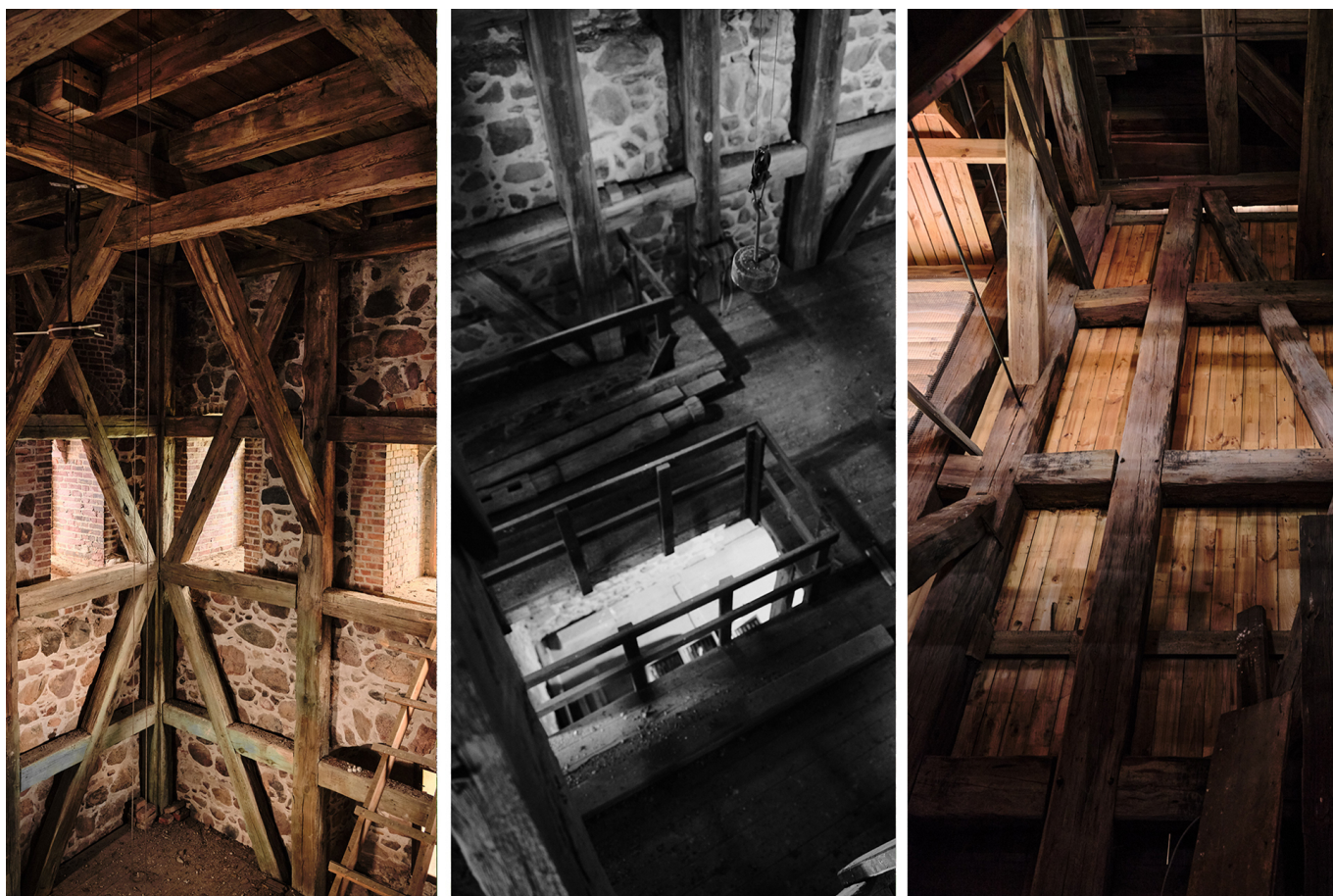
Interior of the church tower, floors 2 and 3 / fot. Aleksander Pukalski / Moryń 2025.
